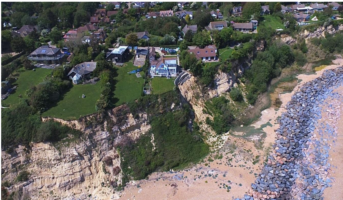
Figures 3.3 (above) and 3.4 (below): In order to preserve the geological interest of the cliffs at Fairlight Cove the rock berm was not set directly against the base of the cliff. This means that an element of erosion and weathering will continue to occur. This can lead to shallow slides and rockfalls particularly after long, wet periods. Following completion of the first two phases of coast protection there remained an undefended vulnerable gap in the defences between the two rock berms. With the assistance of grant aid and partnership funding provided by the Parish Council and Fairlight residents the stage three 250 long berm scheme was completed in early 2017 thereby providing a significantly higher level of coast protection for the whole village frontage.
