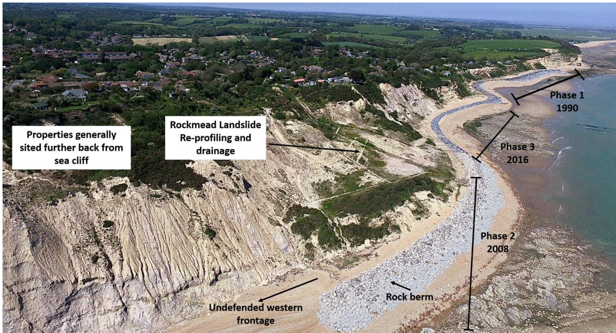
Figures 3.3 (above) and 3.4 (below): In order to preserve the geological interest of the cliffs at Fairlight Cove the rock berm was not set directly against the base of the cliff. This means that an element of erosion and weathering will continue to occur. This can lead to shallow slides and rockfalls particularly after long, wet periods. Following completion of the first two phases of coast protection there remained an undefended vulnerable gap in the defences between the two rock berms. With the assistance of grant aid and partnership funding provided by the Parish Council and Fairlight residents the stage three 250 long berm scheme was completed in early 2017 thereby providing a significantly higher level of coast protection for the whole village frontage.
